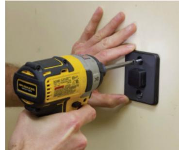
4. Now align the Wall Mount Screw (B) vertically and screw in a second Wall Mount Screw (B) into the wall stud until tight.
